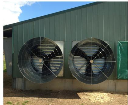
Since the installation of the efficient direct drive fans, there has been no need to replace any fan belts. The new fans have no parts which require maintenance and are highly efficient, so the old belt-drive fans are used infrequently.
