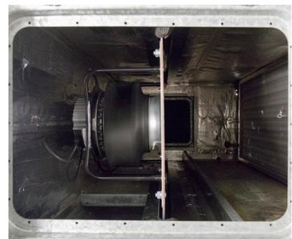
The fan replacement resulted in a more reliable and safe operation of the fume cupboard.
