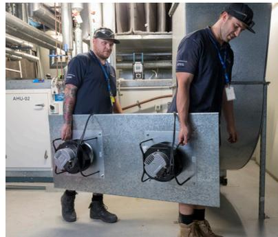
The existing fans, which were speed controlled via VSD, were unreliable, difficult to service and slow to ramp up. The upgrade aimed at improving reliability, unit responsiveness and serviceability.
