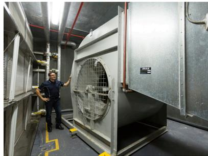
When the original design for the HVAC upgrade, consisting of the replacement of six air-handling units, was put to tender, it specified fewer and larger EC plug fans. In a review of the project, the option to select a smaller individual fan size (500mm instead of 630mm) was put forward by ebm-papst.
